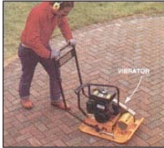
14. TAMP THE PATIO with a flat-plate vibrator after the pavers are installed. Tamp entire outside edge first, then circle in.
