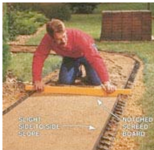
SMOOTH AND LEVEL the sand using a notched screed board riding along the edging for a guide. Include a slight tilt for good drainage.
