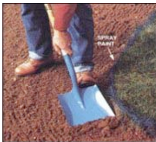
2. REMOVE SOD in an area extending 8 inches beyond the boundaries of the patio. Spray paint indicates the excavation line.
